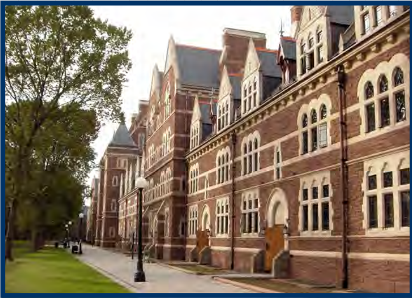
Photo courtesy of Consigli Construction Co., Inc.
